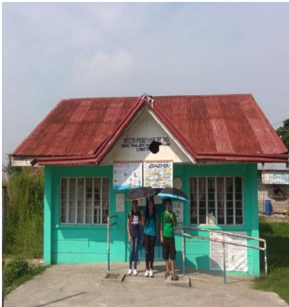
A. Brgy. Tinajero Multi-Purpose Hall
